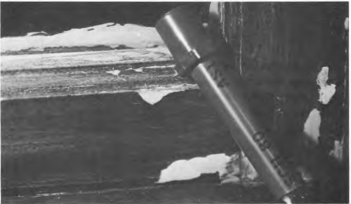
Fig. 18-22. From a basement window, the light sensor keeps track of day and night.
