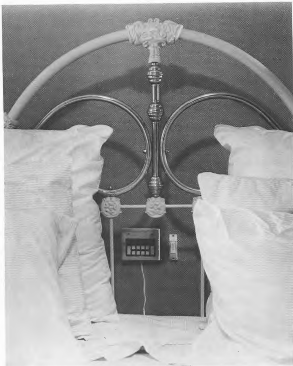
Fig. 18-20. X-10 Controller and panic/emergency button conveniently located in the master bedroom.
